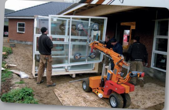
The wide tires make the lifting device suitable for difficult off-road jobs.
